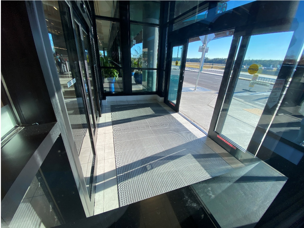
Existing Grates at Airport Terminal Entry Doors
